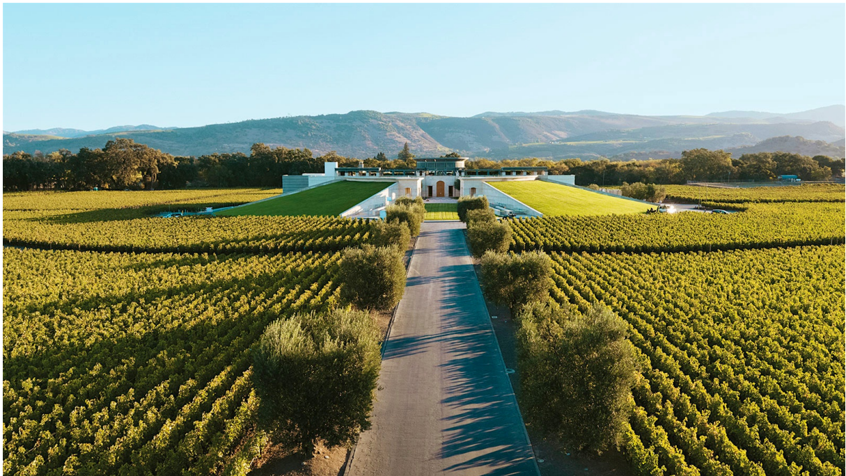
The Opus One winery opened in 1991, with a design that blended neoclassicism with modernity. (Courtesy of Opus One)
